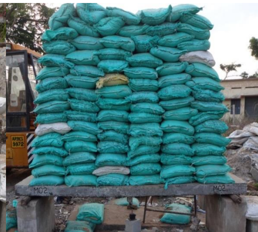
Fig.8 Test load with sand bags for slab MO2
