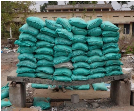
Fig.5 Test load with sand bags for slab MI1
